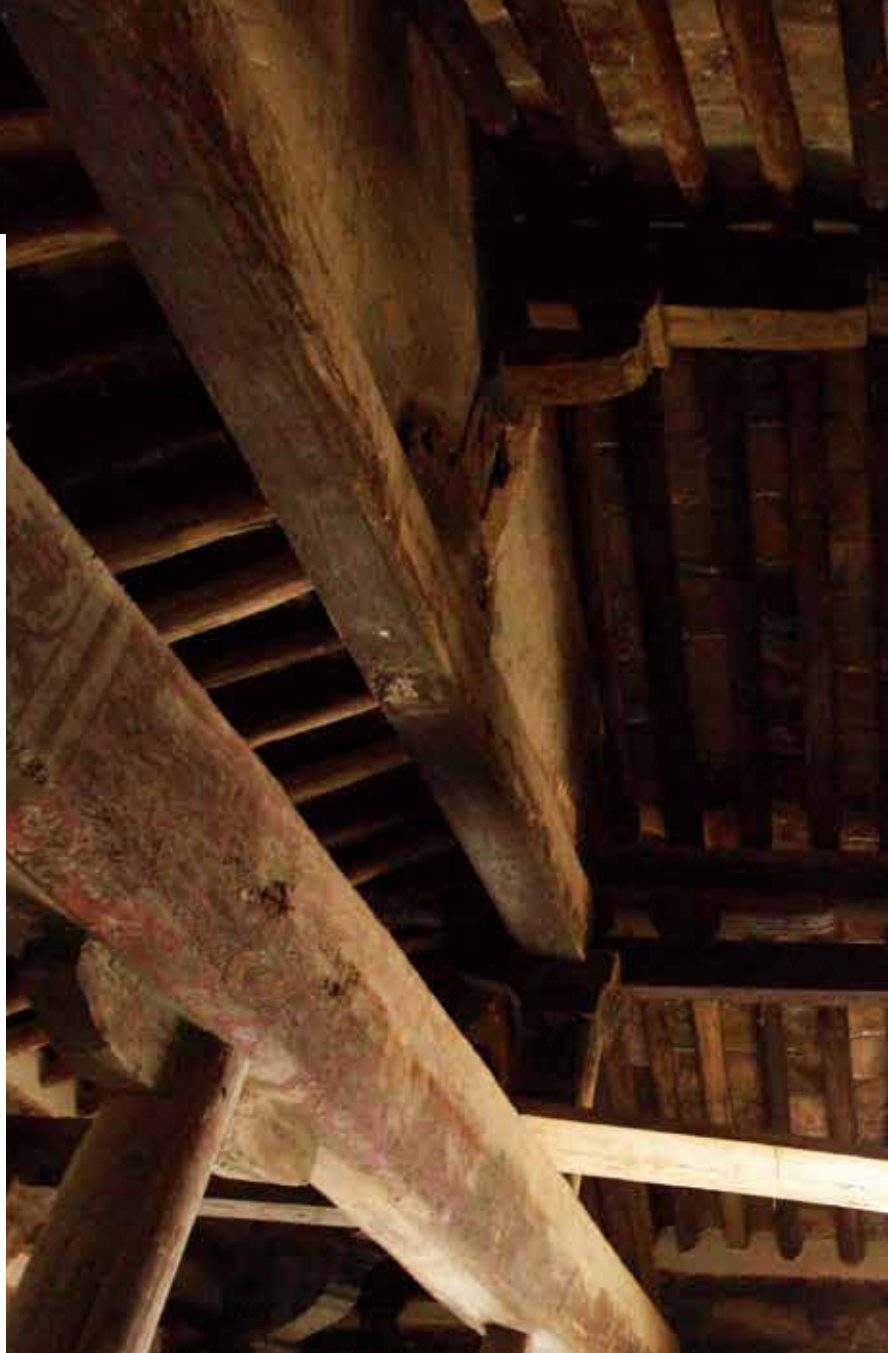
Dou-Gong brackets in Nanchan Temple. Ancient timber-framed buildings in China are usually built with Dou-Gong brackets and sockets to connect all posts and beams, without any metal connectors like nail, screw, or bolt.
