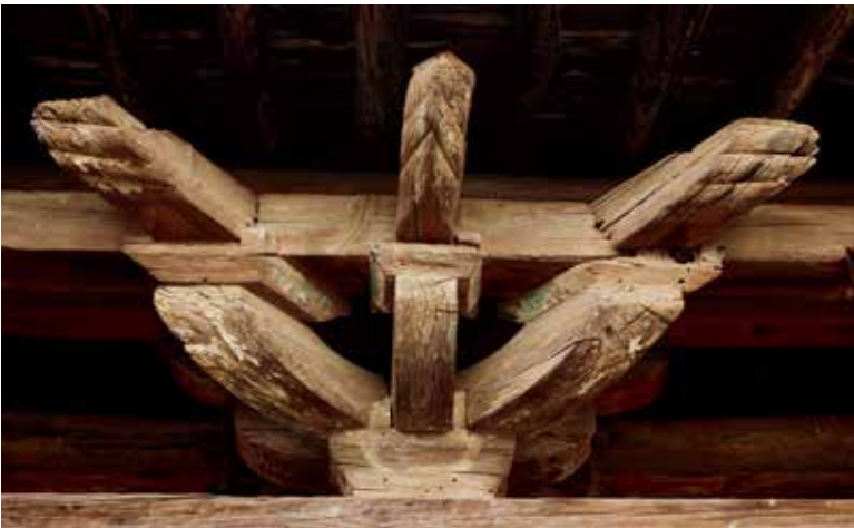
Dou-Gong brackets in Nanchan Temple. Ancient timber-framed buildings in China are usually built with Dou-Gong brackets and sockets to connect all posts and beams, without any metal connectors like nail, screw, or bolt.
